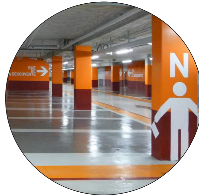
Parking souterrain Le Ruban Bleu_St Nazaire
